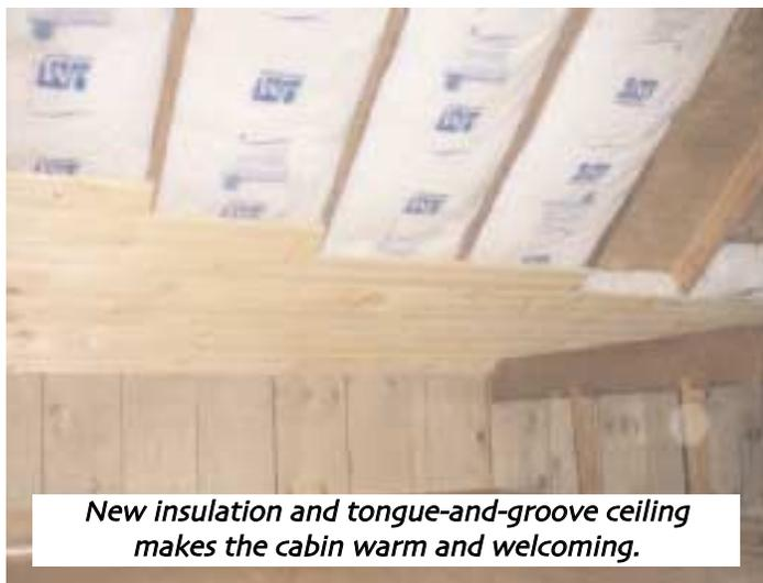
*New insulation and tongue-and-groove ceiling makes the cabin warm and welcoming.*
