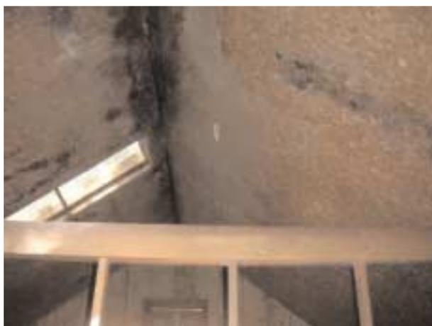
*Much of the interior ceiling was ruined due to moisture, which caused rot and mold.*
